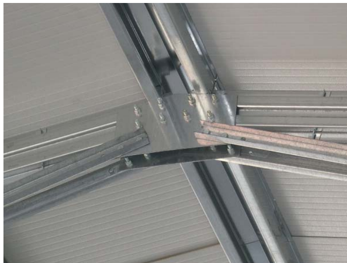
Diagonal bearing structures – truss detail
