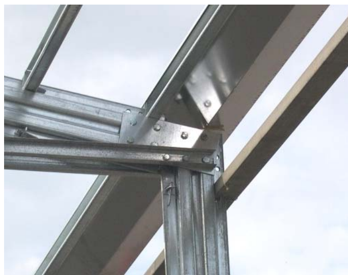
Post – truss detail
