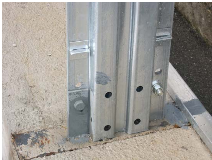
Post – Basement detail
